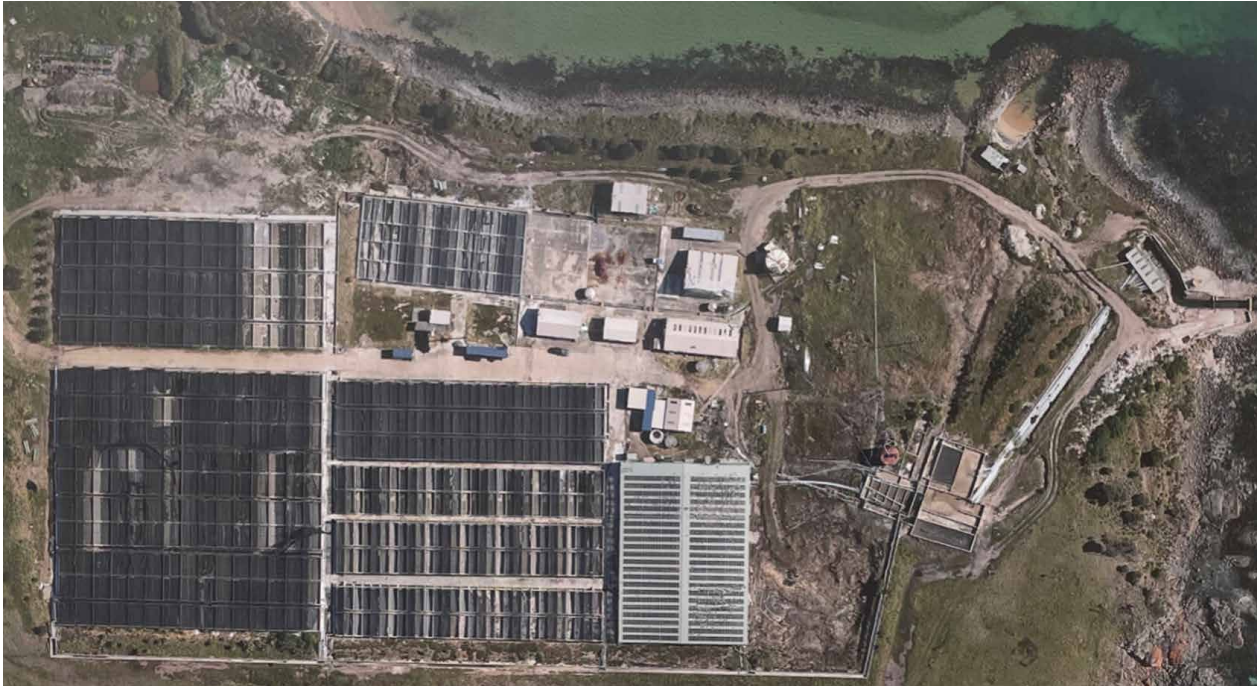
Figure 3.4 – Sea Forest facilities in Swansea, Tasmania
