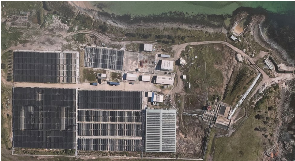
Figure 3.4 – Sea Forest facilities in Swansea, Tasmania
